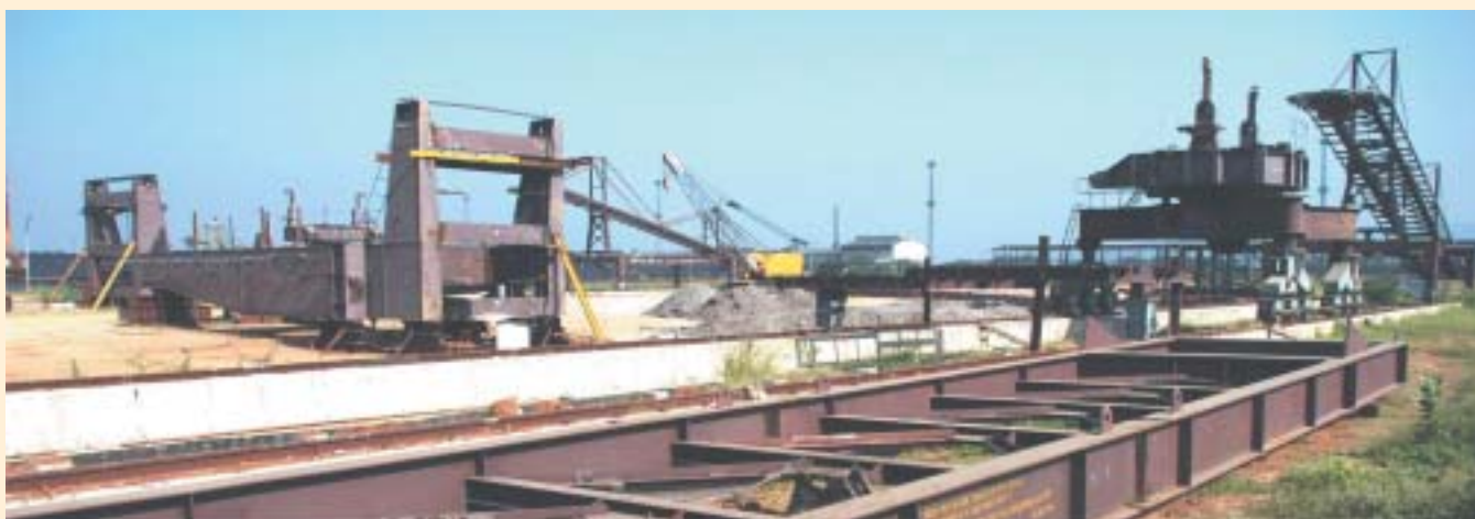
Erection of Stacker-cum-Reclaimer at Vishakhapatnam Steel Plant (RINL).
