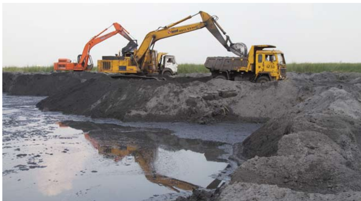
Extraction & transportation of ash from ashpond at Bokaro by HSCL.
